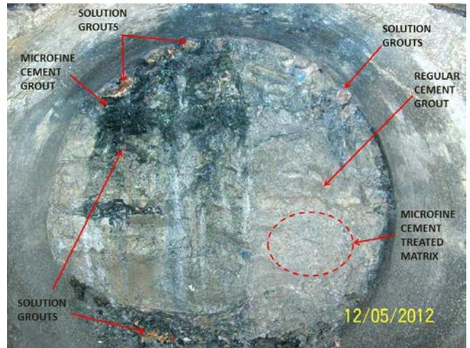
of 500+ gallons immediately flooded the TBM and shaft halting tunnel construction. ECO was again called upon by the Contractor to reduce the water inflow around the TBM to a manageable inflow that would allow for the break-in to occur and the tunnel liner to provide a water seal. This was a formidable grouting challenge because the TBM could not be locked in place with the grout.
