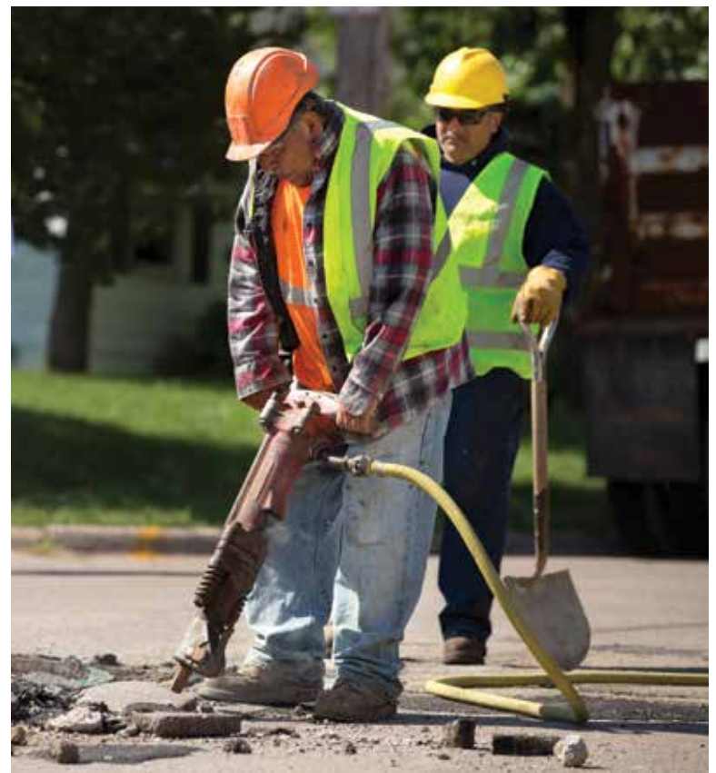
Roberto Lopez jackhammers surface material around a manhole at the start of a rehabilitation project in Davenport, Iowa.
