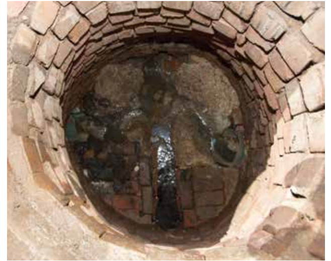
BELOW BOTTOM The manhole after installation of a Reliner channel system.
