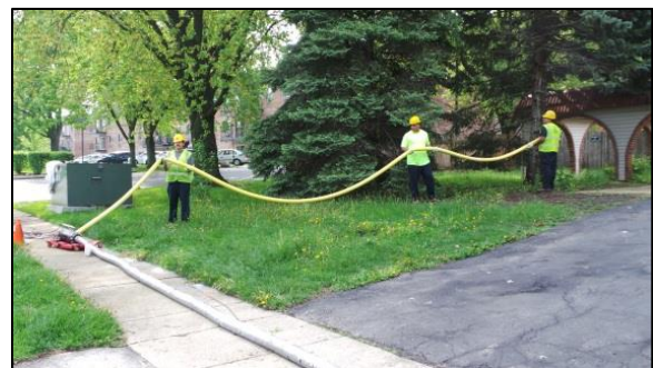
Figure 2. 38 foot lateral sock
