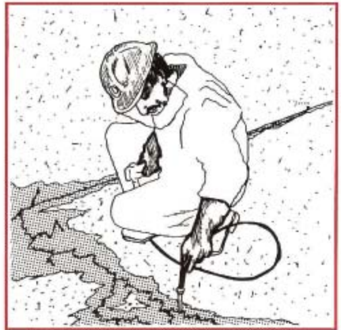
Injection of PUR grout into floor slab crack. Note disposable covers/alls and protective equipment.
